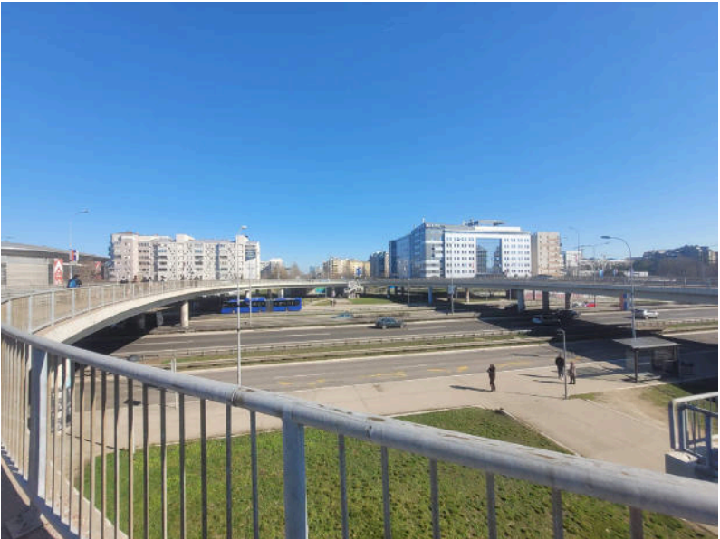
Overpass from the Highway of New Belgrade
